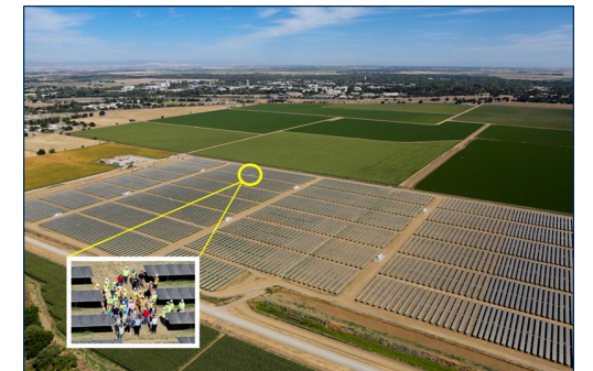
16.3 MW Large Solar Power Plant
