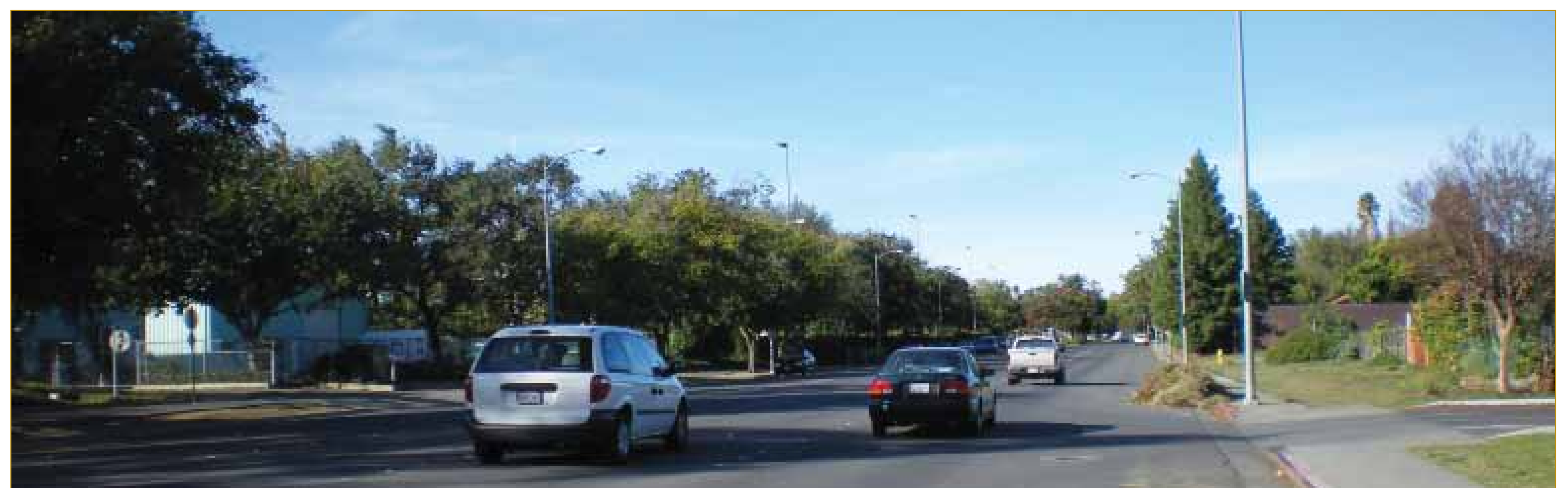
▲ The City of Davis is working to convert a major corridor that currently consists of four vehicle lanes, to a roadway that consists of two vehicle lanes, two bicycle lanes, and enhanced pedestrian amenities.
