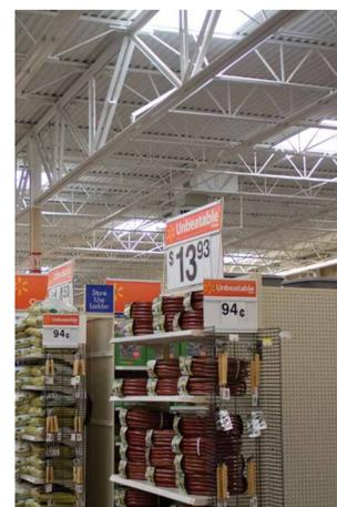
Skylights (above and right) help big-box retail stores use daylight to reduce electric light use. A dual-loop photosensor dimming control system contributes to additional energy savings and reduced maintenance costs.
