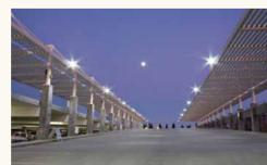
The Smart Lighting Initiative uses efficient lights and sensors to reduce lighting when facilities are vacant. A parking structure near the Mondavi Center features this technology. Once installed in all parking structures the initiative could save 1.3 million kWh annually.
